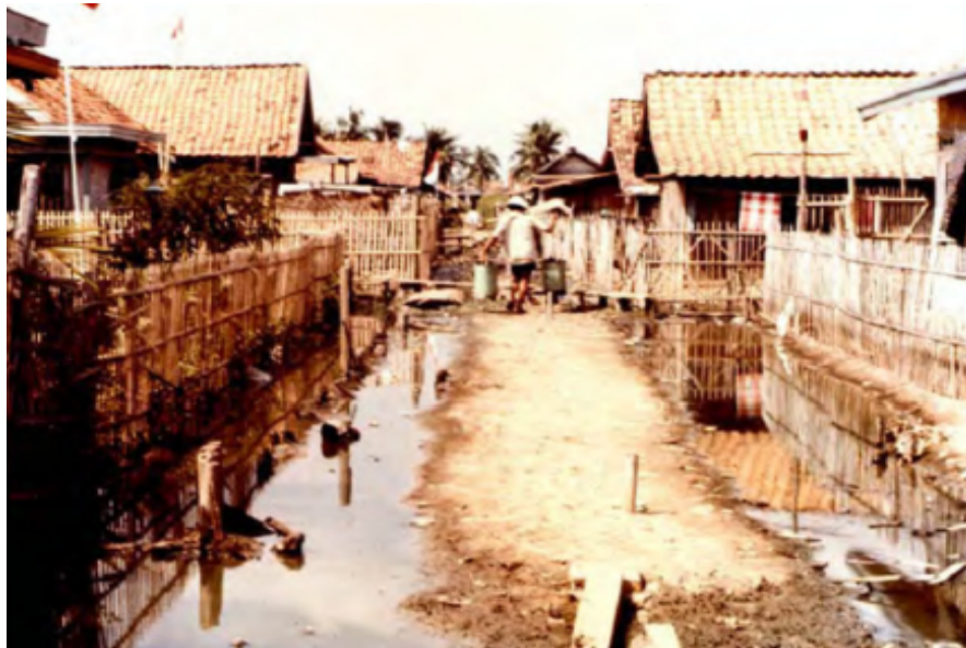
Figure A1: Kampung in Jakarta, before and after KIP ( Darrundono, 2012 )
